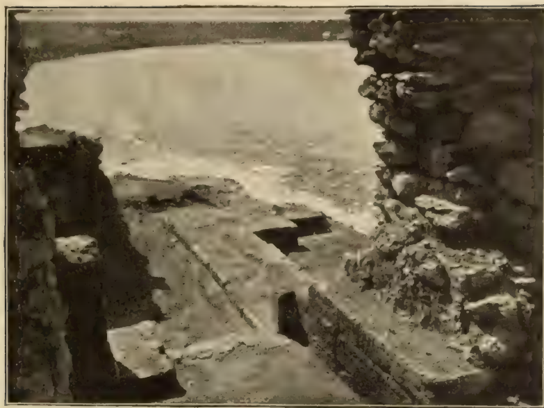
FIG. 336. CR. 1895, p. 103, f. 254. Chersonese. NW. postern \phi with foundation of tower P^2 .
