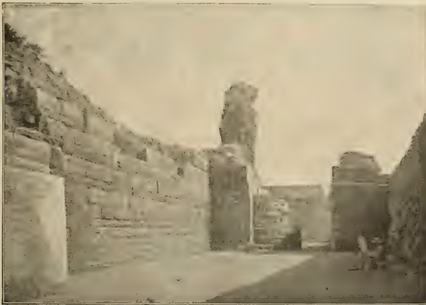
FIG. 335. BCA . I. p. 29, f. 23. Greek walls at Chersonese looking SE. from near c towards Dd . Seven courses of first period, four of second with round tower D . Upper work and square towers Dd , Roman.
